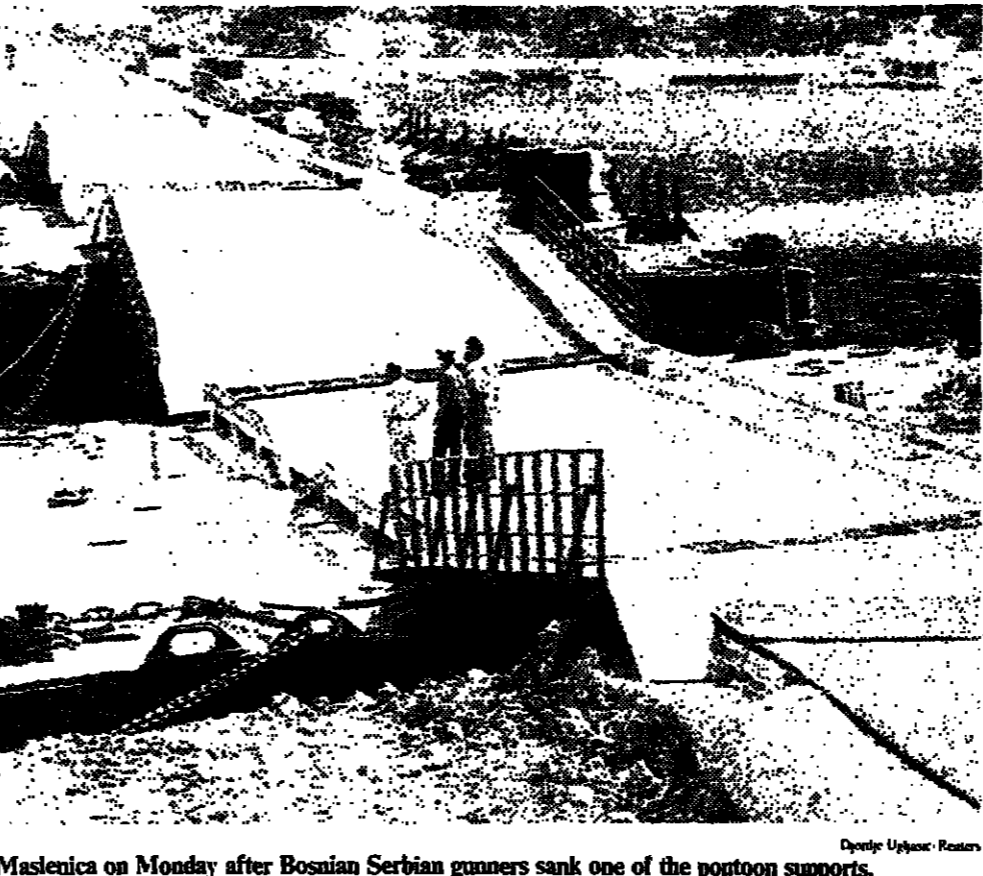
Croatians inspecting a bridge at Maslenica on Monday after Bosnian Serbian gunners sank one of the pontoon supports. (AP, Reuters)
